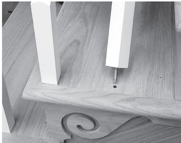
Figure 11 — Using baluster fastener to attach baluster
