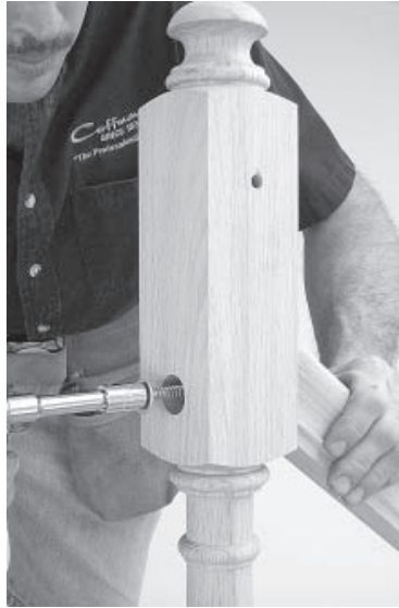
Figure 10 — Attaching handrail with lag screw (bolt) from back side of newel
