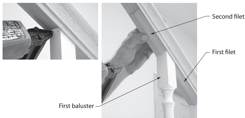
Figure 12 — Nailing a baluster to the handrail
