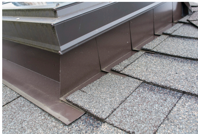
Figure 19 —Typical skylight flashing
