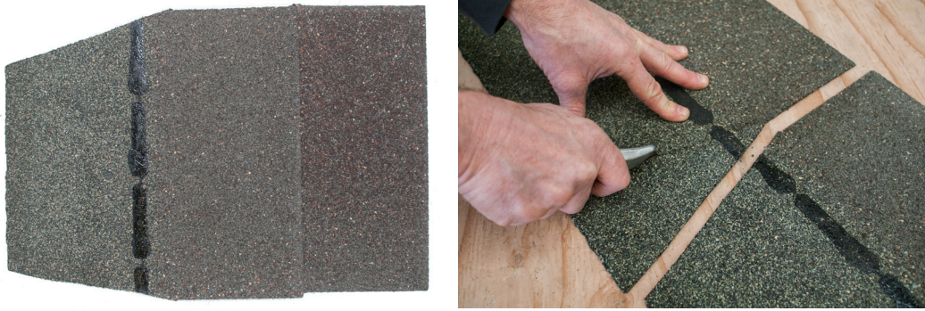
Figure 10—Cap shingle and cutting a cap shingle
