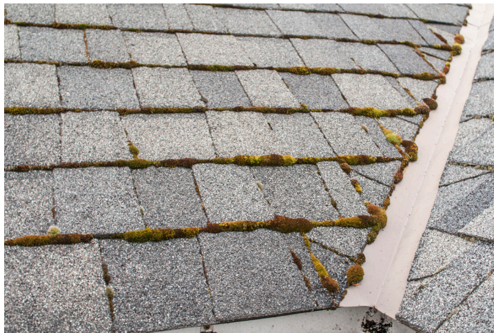
Figure 3—Moss growth on laminated asphalt shingle roof
