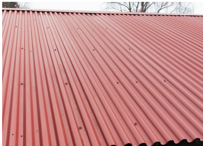
Figure 8 —Sheet metal roofing with exposed fasteners
