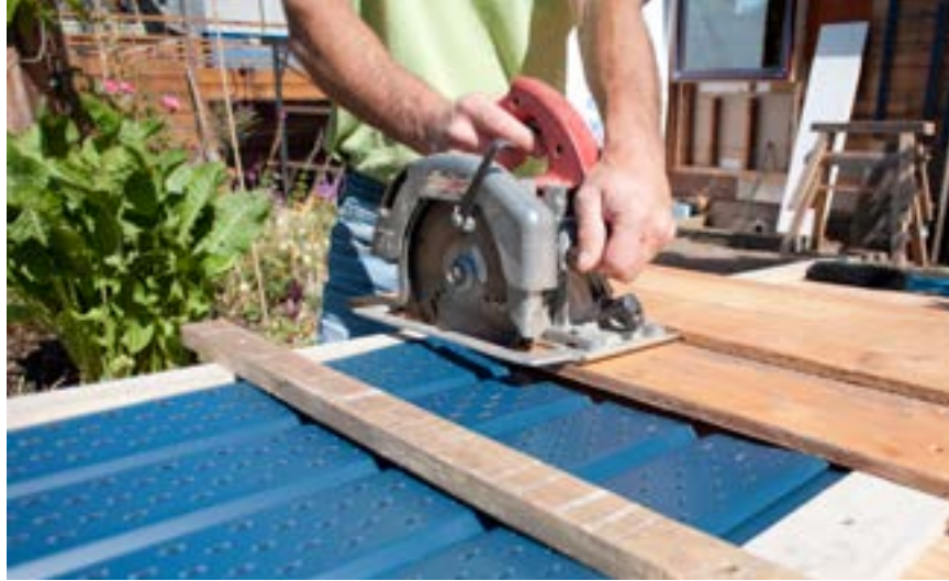
Figure 32—Crosscut jig for siding or soffit
