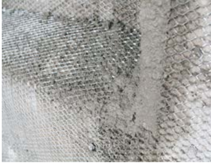
Figure 43—Expanded metal lath reinforcing the corner
