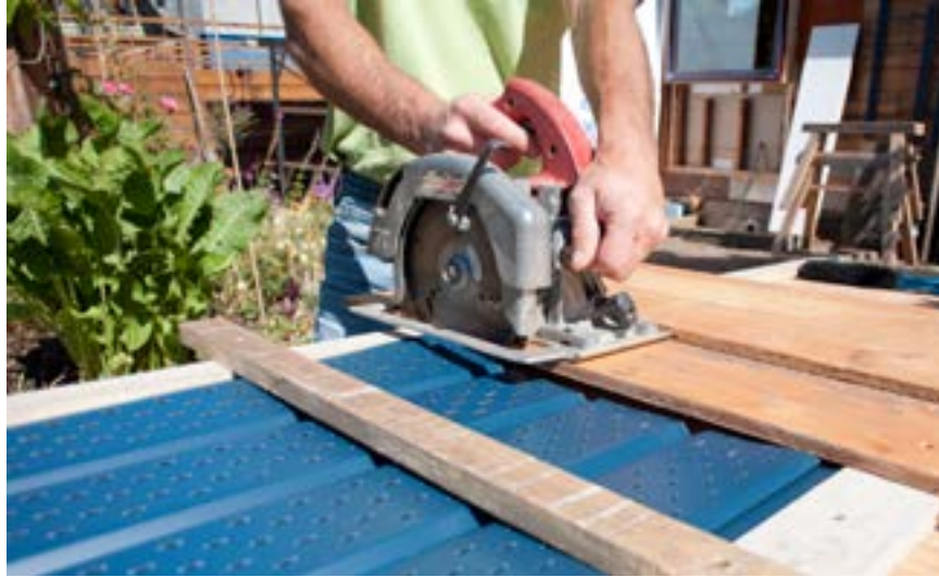
Figure 15—Cross cut jig for siding or soffit
