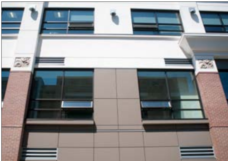
Figure 5—Example of a panellized EIFS
