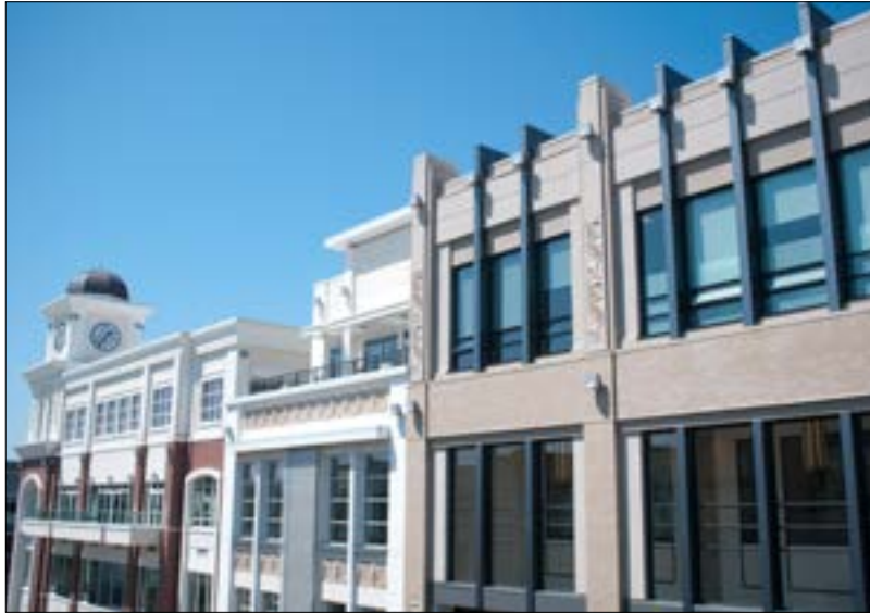
Figure 4—Example of an EIFS
