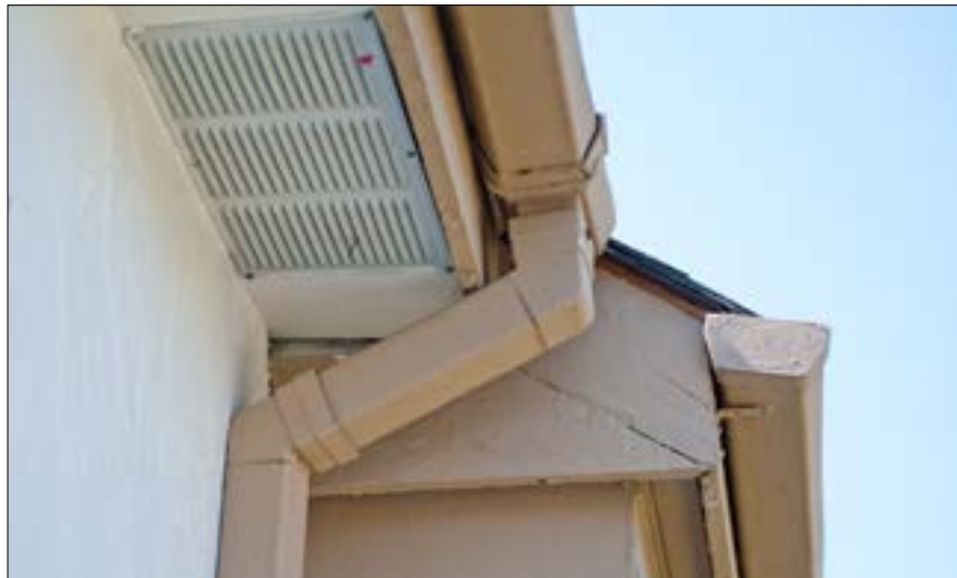
Figure 70—Examples of a vinyl gutter. Two elbows offset the downspouts to the wall.
