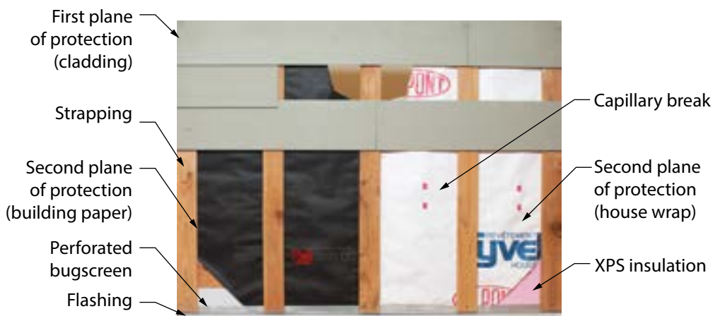
Figure 1—Components of a rainscreen wall
