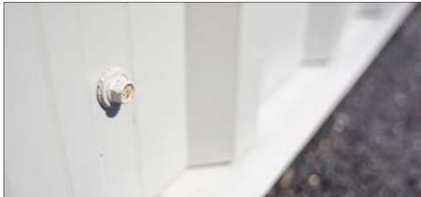
Figure 10—Sheet metal siding with fasteners
