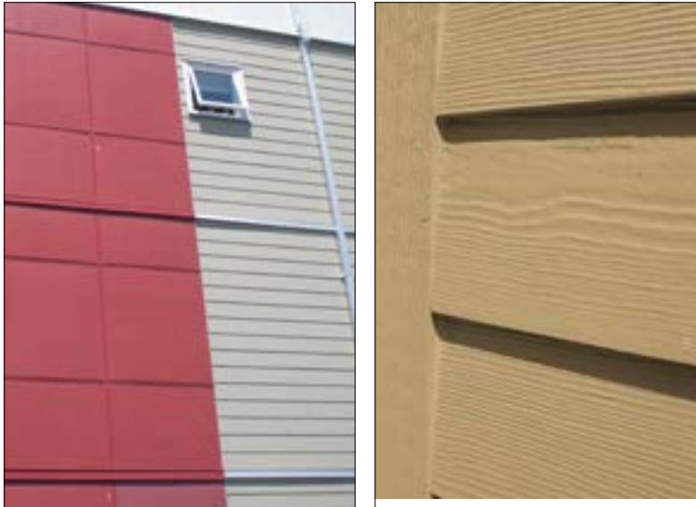
Figure 11—An example of fibre cement panels (left) and textured lap siding (right)
