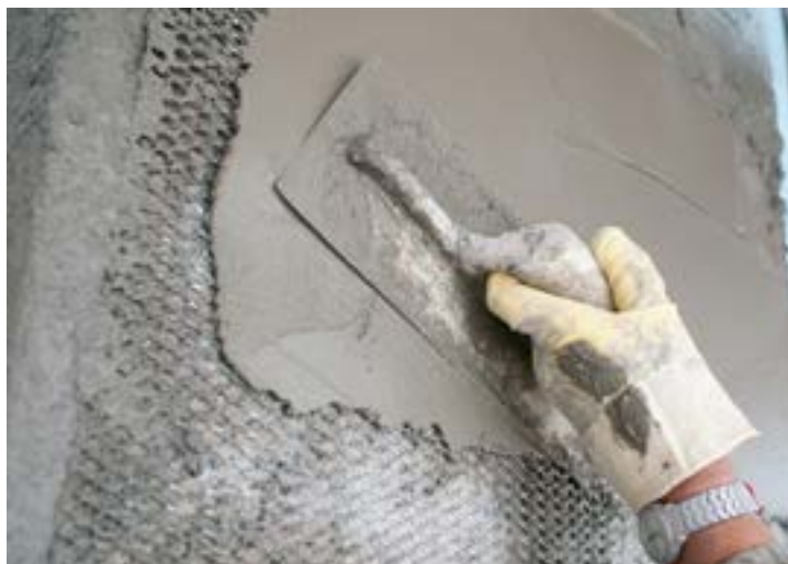
Figure 7—Stucco over expanded metal lath
