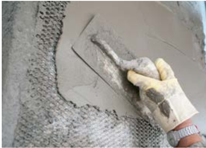
Figure 42—Stucco over metal lath
