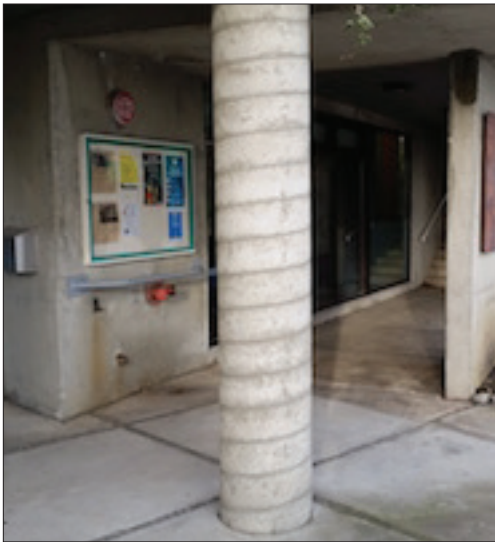
Figure 12 — Column formed with unlined cardboard
