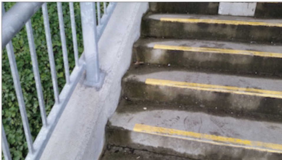
Figure 18 — Embed for handrail attachment
