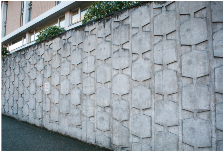
Figure 3 — Finishes achieved with form liners
