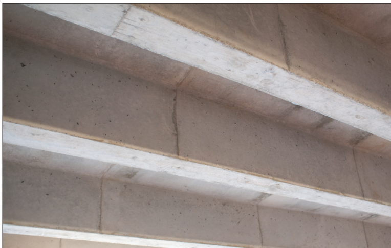
Figure 10— Concrete ceiling created with dome pans
