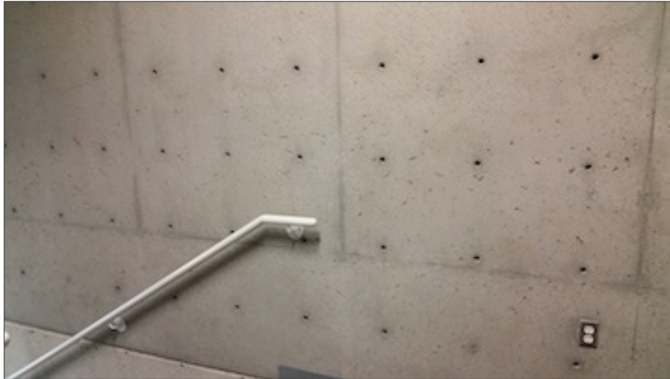
Figure 1 — The result of tight, properly aligned seams
