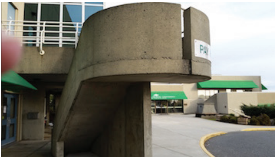
Figure 16 — 5-foot-radius curved wall
