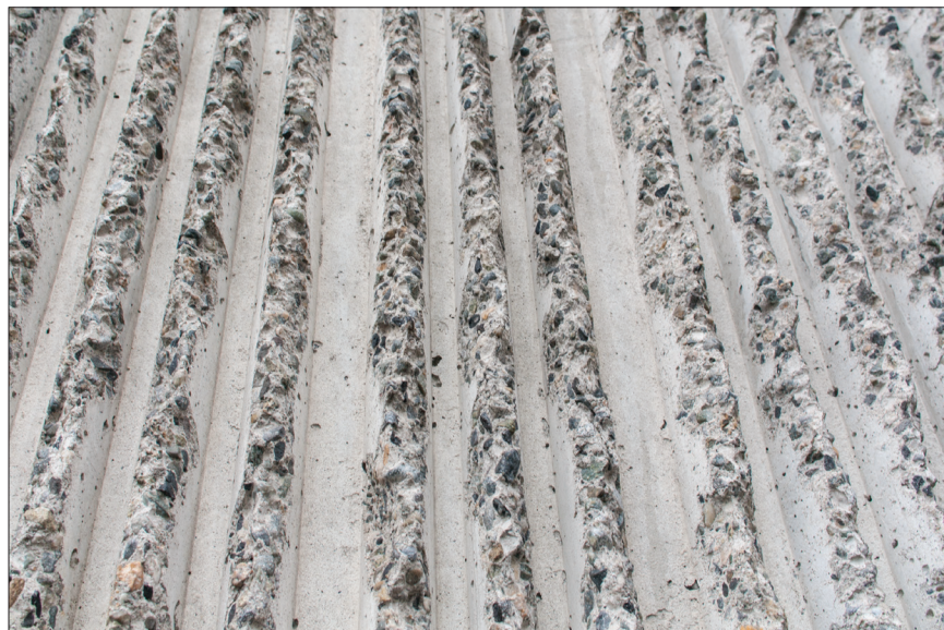
Figure 5 — Broken fin (fractured) finish
