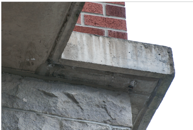
Figure 11 — Reveal acting as a drip
