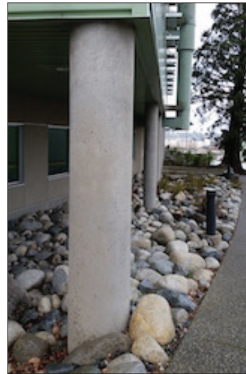
Figure 13 — Column formed with two-piece metal form
