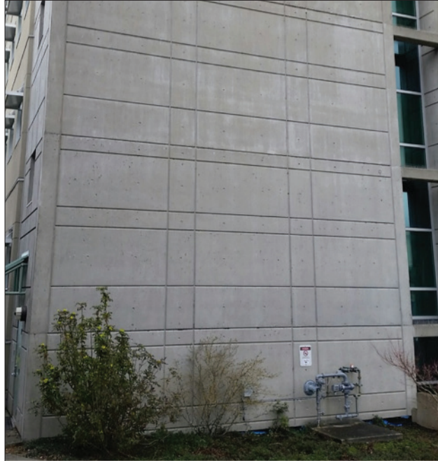
Figure 7 — Wall with rustication strips used to hide both sheathing joints and construction joints
