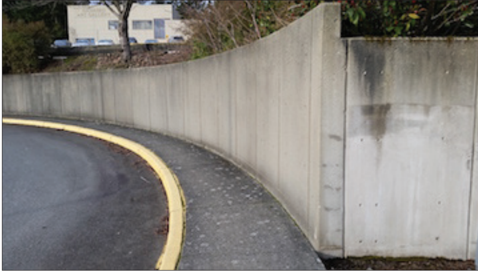
Figure 15 — 60-foot-radius curved wall
