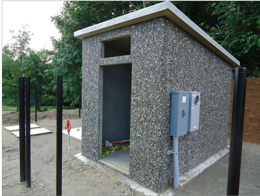
Figure 4 — Exposed aggregate vertical finish
