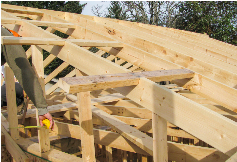
Figure 21 — Notched rafter supporting outriggers
