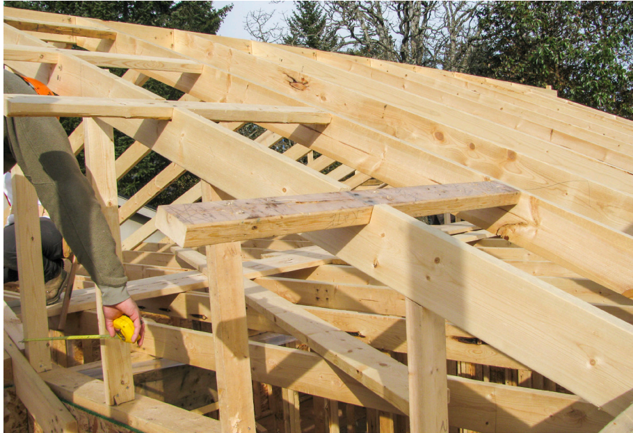
Figure 9 — Outriggers notched into gable rafter
